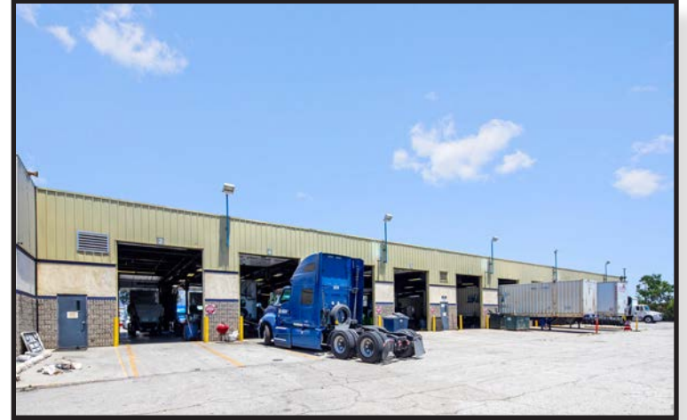
South Side of Shop
