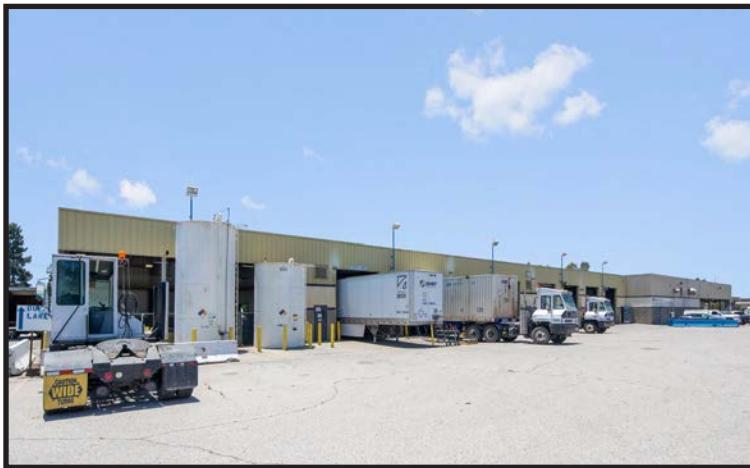
North Side of Shop
