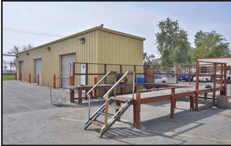
Fire Sprinklered Storage Building
